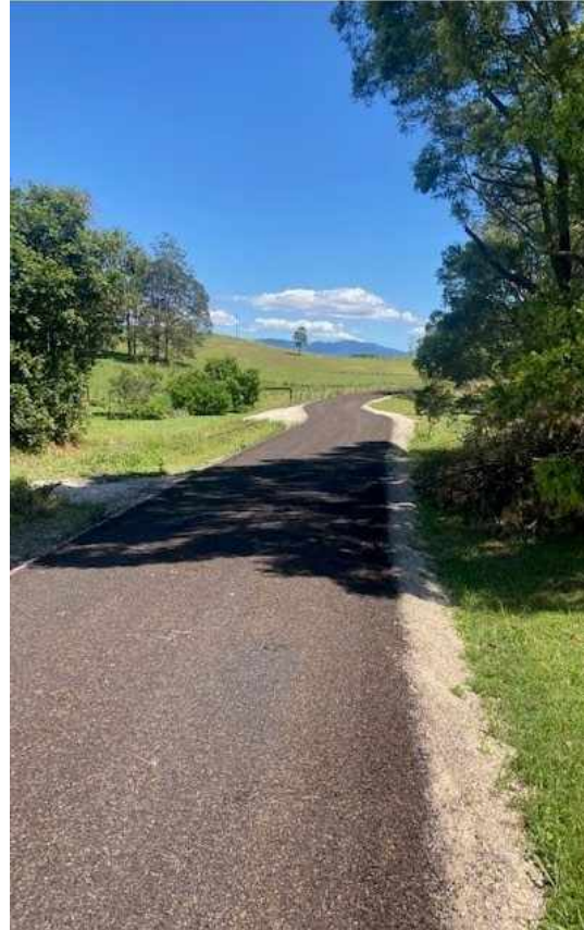
Stokers Siding – facing north
