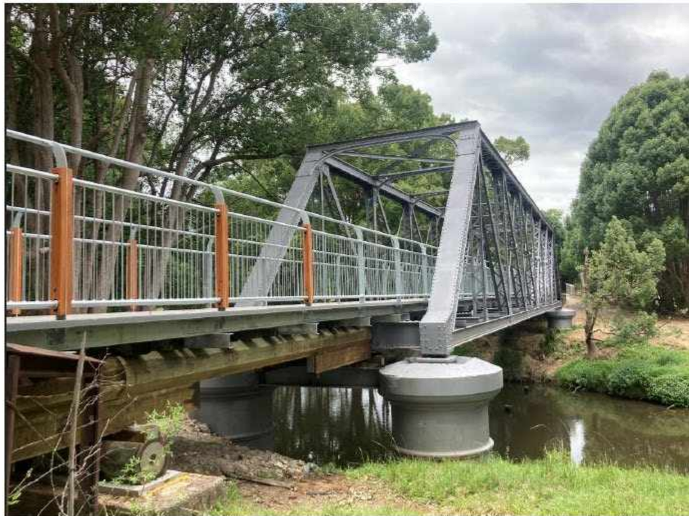
B15_01 refurbishment 100% completed as of 31 December 2022
