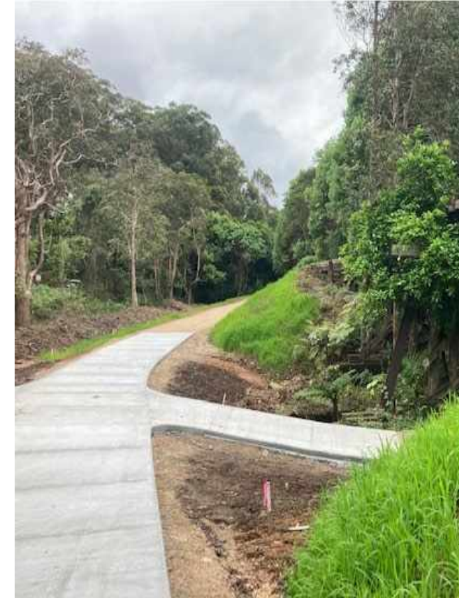
Crabbes Creek – B22_01 bypass, facing north
