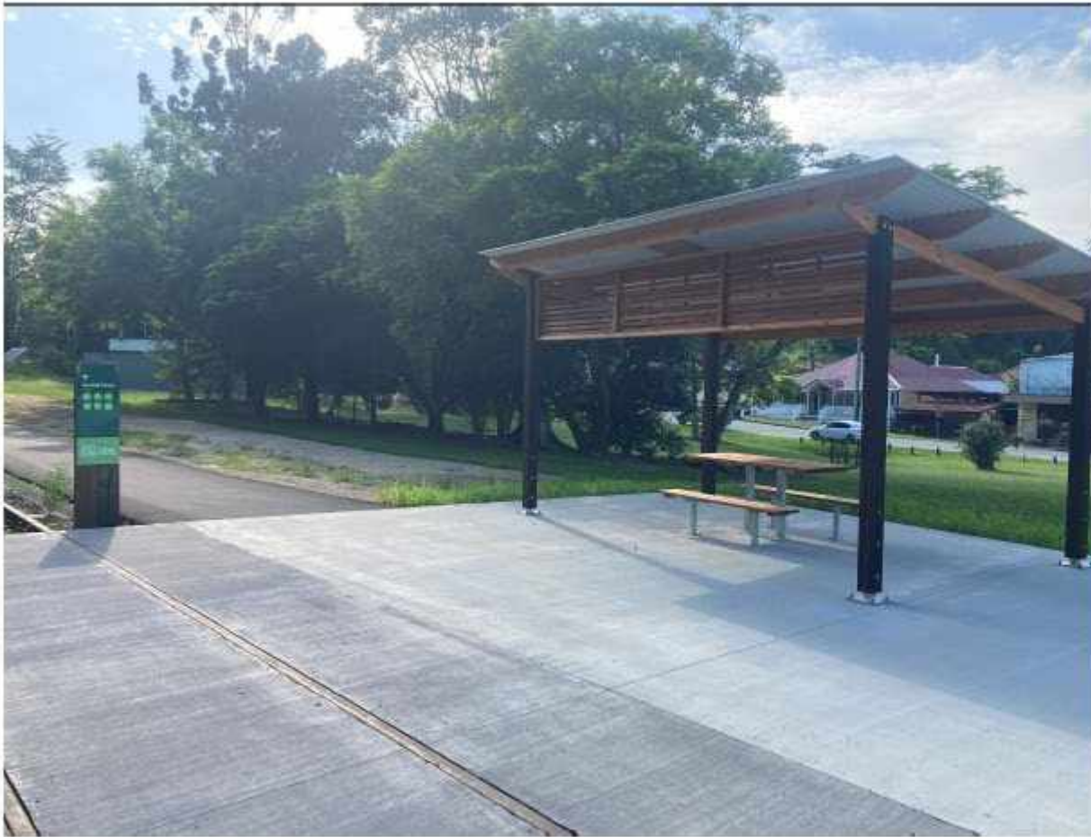
Burringbar heritage station – completed works December 2022
